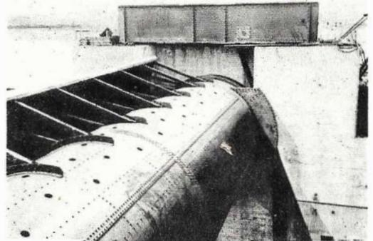
A view of the roller-gate dam at Canton, Mo. Just behind the steel gate is the concrete piece in which are installed 6 mammoth water heaters; these melt ice around dam in winter.
