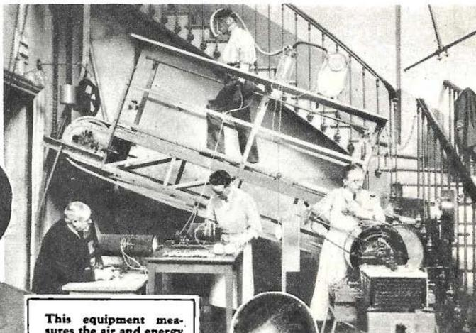
This equipment measures the air and energy a human "guinea pig" consumes in walking continuously up moving floor at the rear.
