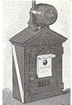
The siren at top of this fire alarm box sounds for one minute when handle is pulled, to discourage vandals from ringing false alarms.
