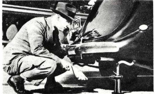
This extension bolted to the chassis side members at both front and rear provides an accessible jack rest on streamlined cars. Tire changing is much simplified by this improvement.
