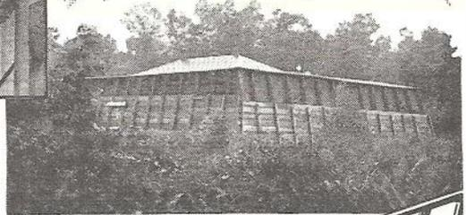
The roof of this isolated dynamite packing house can just be seen over the top of the heavy timber barricade used to divert the force of explosion upward.
