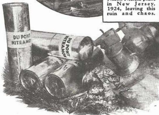
This new explosive, known as Nitramon, is immune to flames, and can be detonated only by a large charge of dynamite. Large supplies of Nitramon can be stored in safety, where ordinary stick dynamite or TNT would prove too hazardous.
