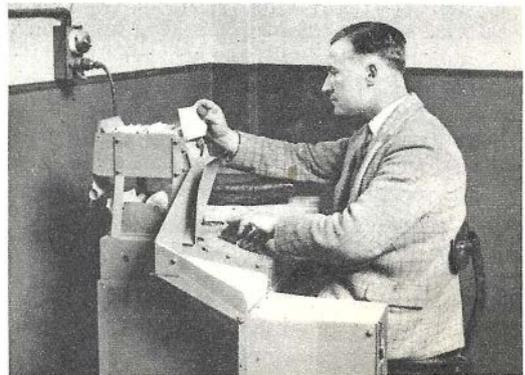
This robot letter sorter is operated by a keyboard on which the principal cities are designated by number. It is only necessary to press the required button and the letter is pouched.
